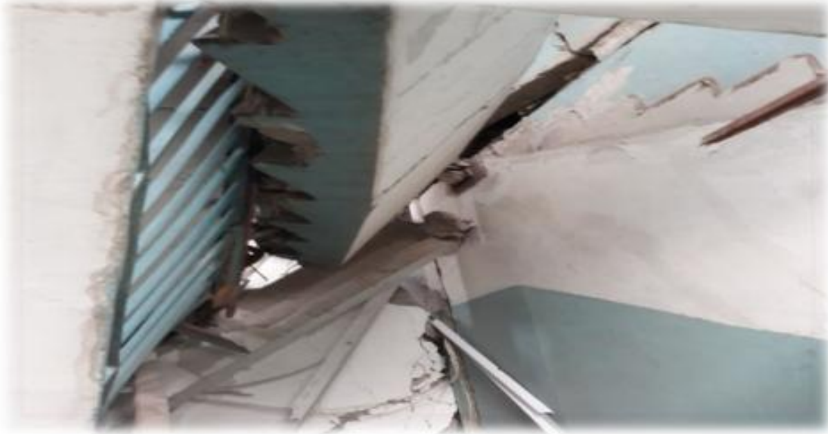
The stairs that collapsed from the aerial bombardment in the corridor of my house. Mariupol. March 2022. Photo by Maria Saraieva.
