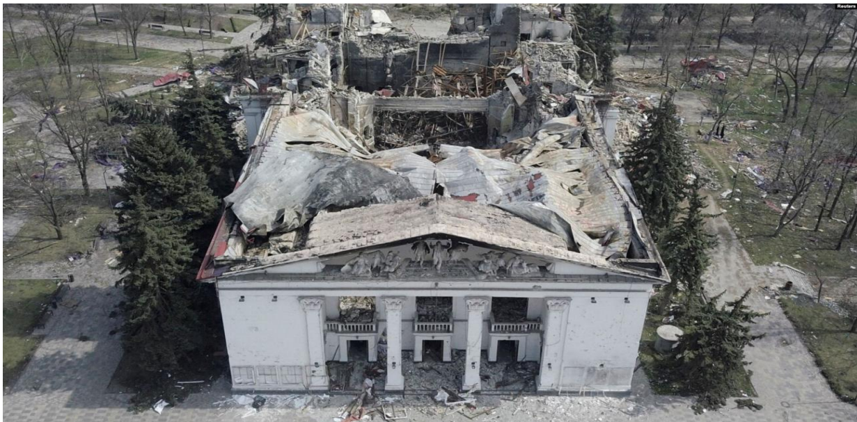
Mariupol regional drama theater. Destroyed. March 16, 2022.
