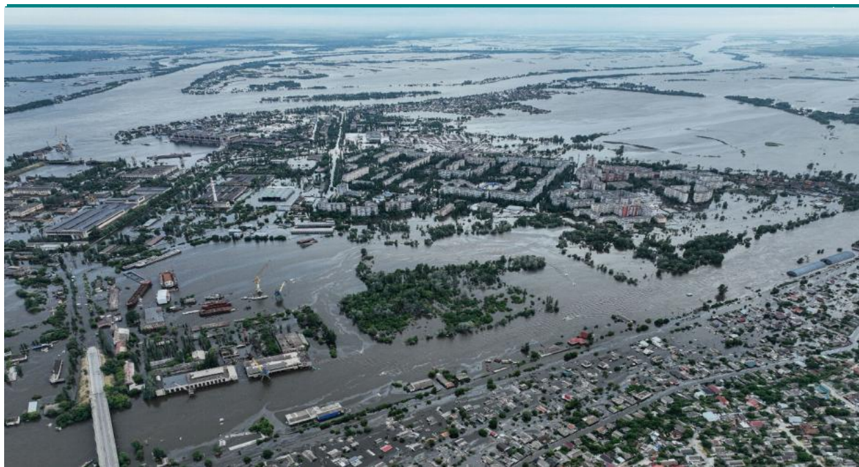
The collapse of Ukraine's Nova Kakhovka dam. June, 6, 2023.
