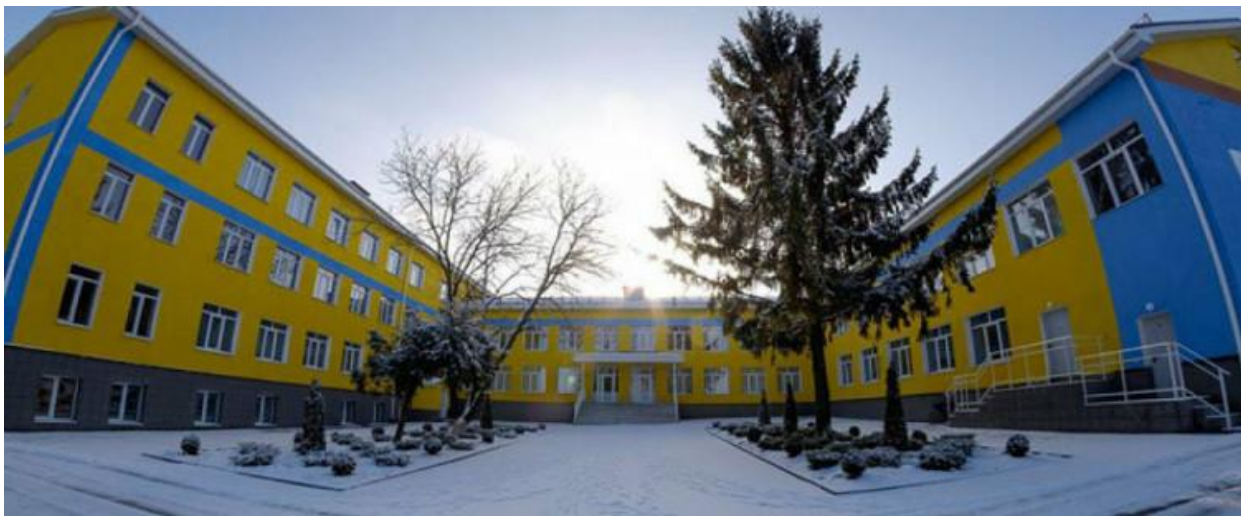
Renovated school No. 5 in Volnovakha before the russian invasion. 2020. Photo: Volnovakha.City. Donetsk Regional State Administration. https://dn.depo.ua/ukr/dn/yakoyu-bula-volnovakha-do-viyini-rosiyska-armiya-znishchila-misto-za-dva-tizhni-202203131433577 (Revised: 10.07.2024)
