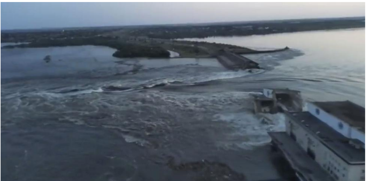
Water leakage from the Kakhovka Reservoir due to a destroyed dam. June 6, 2023. Reuters. https://www.radiosvoboda.org/a/pidryv-kakhovska-hes-evakuatsiya-zahroza-zaes/32446581.html (Revised: 10.07.2024)
