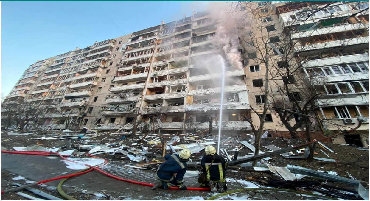
A house in Kyiv in Podilsky District after russian shelling. 15.03.2022. Author: State Emergency Service of Ukraine. Source: https://www.facebook.com/photo/?fbid=332944558873440&set=pcb.332944848873411 (Revised: 10.07.2024)
